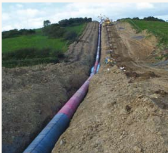
Trenching in Agricultural Land
