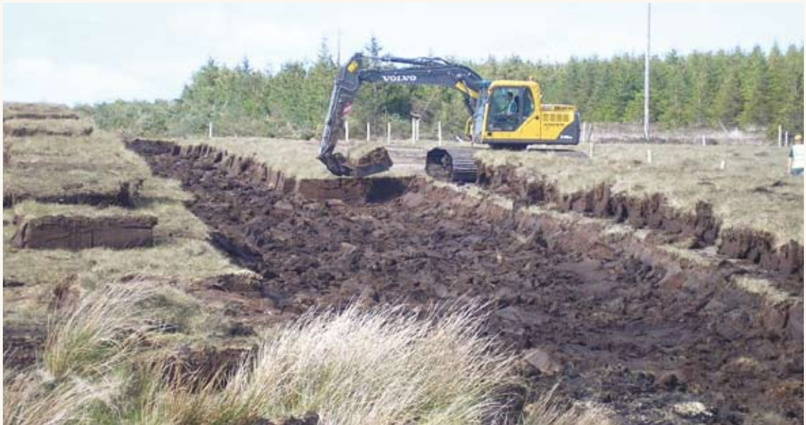
Preparation for Construction of Pipeline in Peatland (Mayo-Galway Pipeline, 2006)
