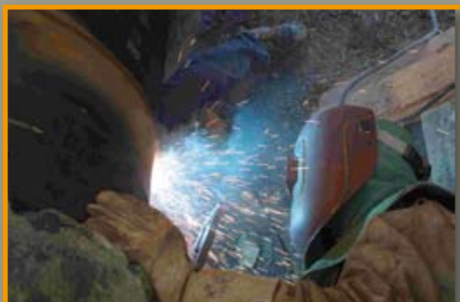
Manual welding in process
