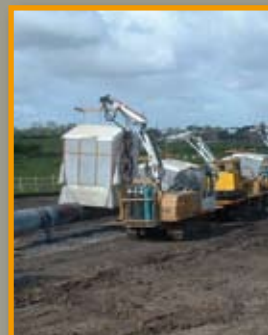
“Train” of automatic welding each completes one weld p
