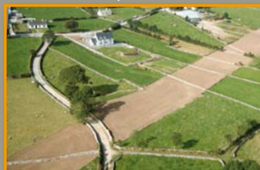
Reinstatement on section of Gas Pipeline to the West in Co Galway
