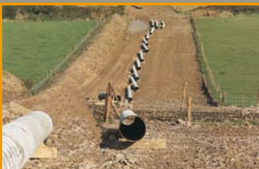
Pipeline sections laid out and ready for welding
