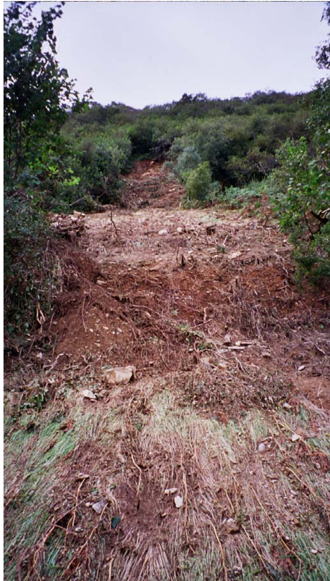
Figure 4.2 Views Looking Up Landslide Debris Trail
