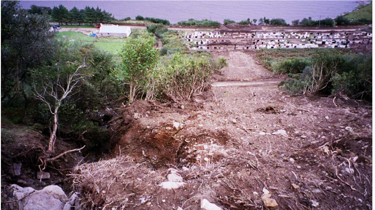
Figure 4.1 View Looking Down Landslide Debris Trail
