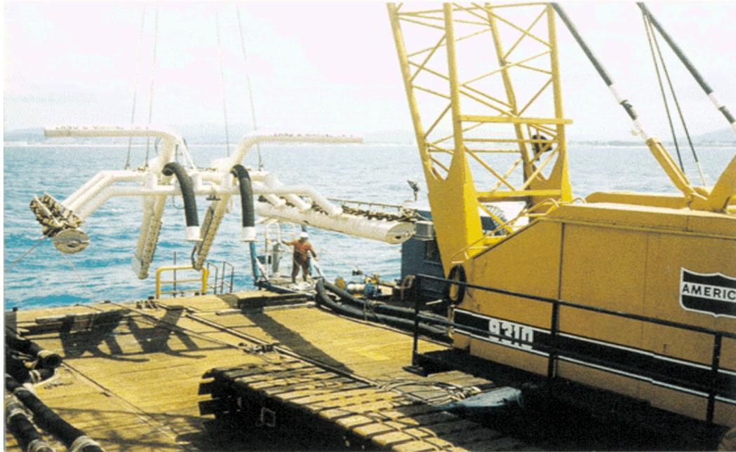
Plate 3.4: Typical inshore sediment “jetting” equipment
